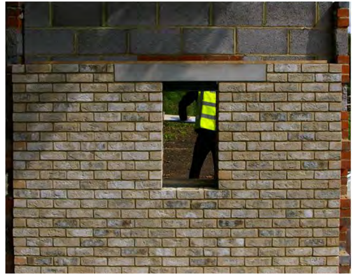
June 2019: Internal facade of sample panel
