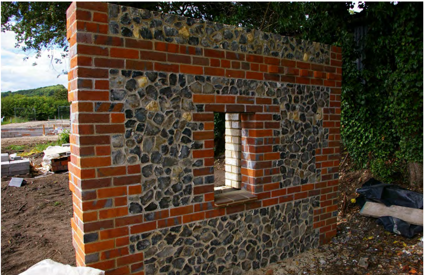
June 2019: Sample panel on site
