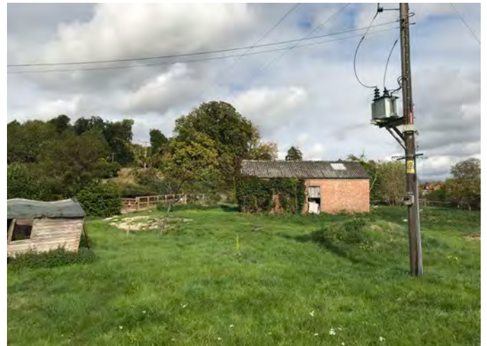
View 2: 1950s outbuildings and timber pylon
